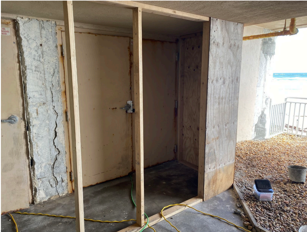
Picture 3: In-progress hardwall installation
