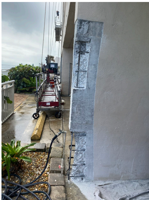
Picture 2: Completed excavations
